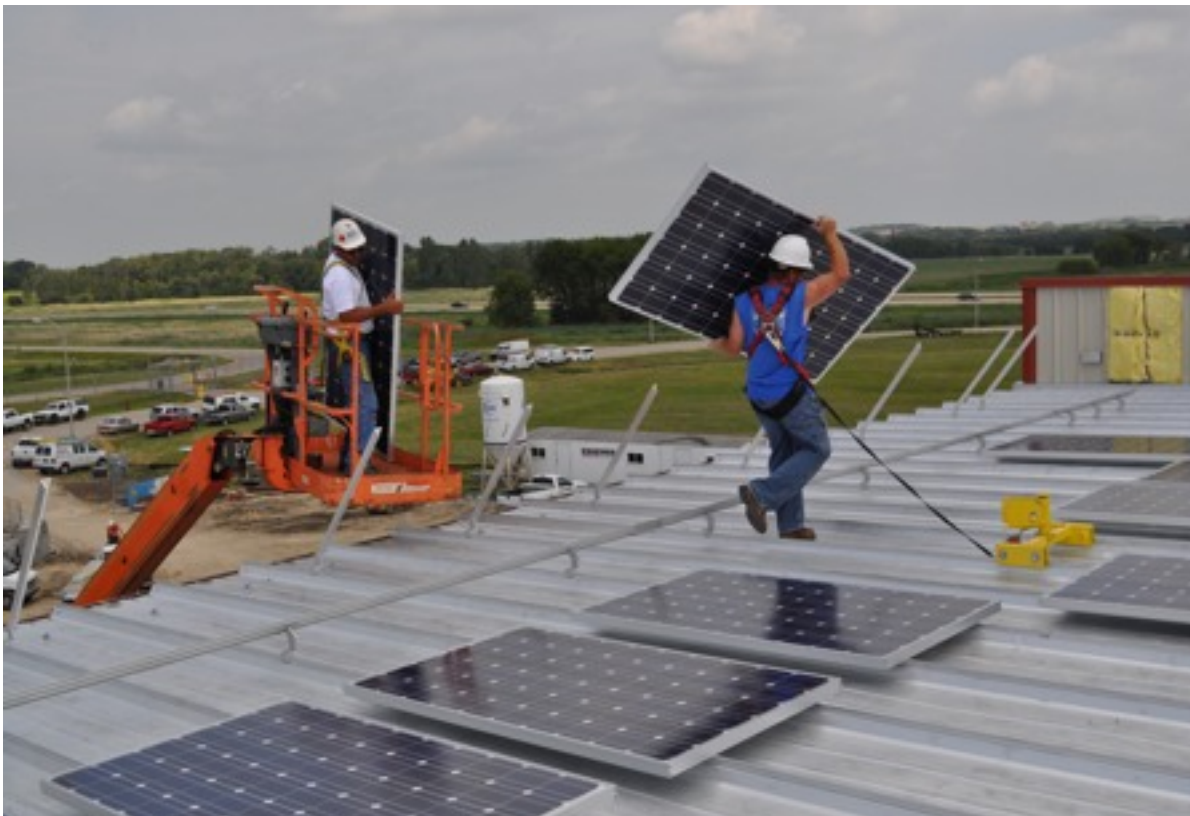
Courtesy and Copyright H&H Solar Energy Services Madison, Wisconsin
